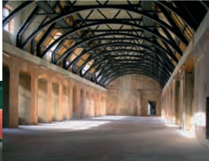
The "Riesensaal" in the Palace (east wing, 2 nd floor), condition in 2007
