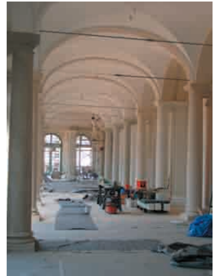
Construction work for the new Oriental Gallery in the Zwinger
